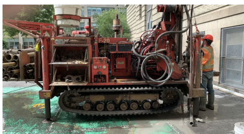
Drilling on site to analyze the soil condition
